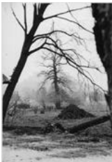
BLICK VON DER HOFHAY- MER ALLEE IN RICHTUNG FESTUNG VIEW FROM HOFHAYMER ALLEE TOWARDS THE FORTRESS
